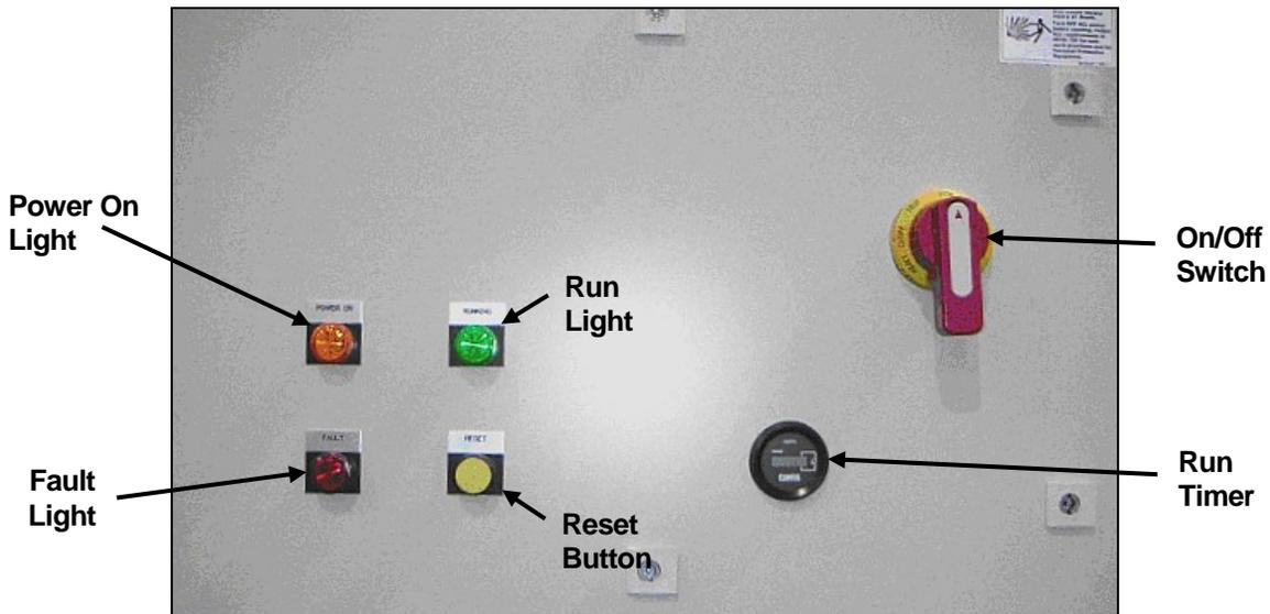
**Figure 7. Gas Pack Control Console Panel**
